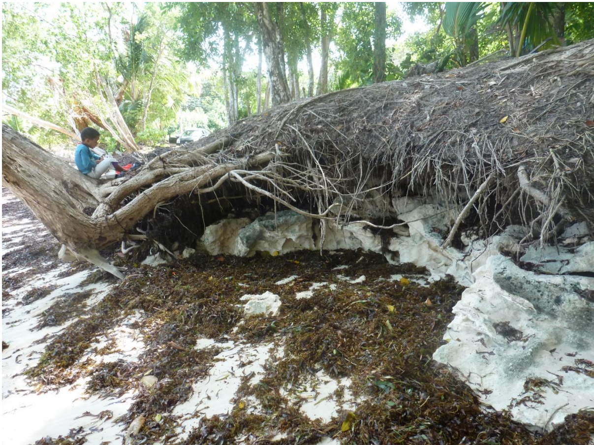
Fig. 1a. Severe beach erosion is common along the coastal zones in the Seychelles
